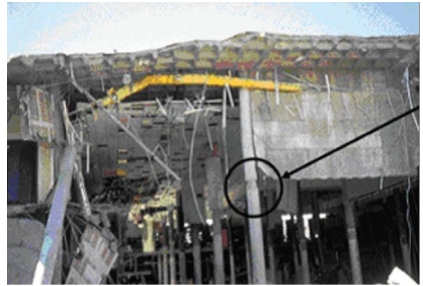
Figura 5. Falla por punzonamiento (Journal of engineering and technology)
