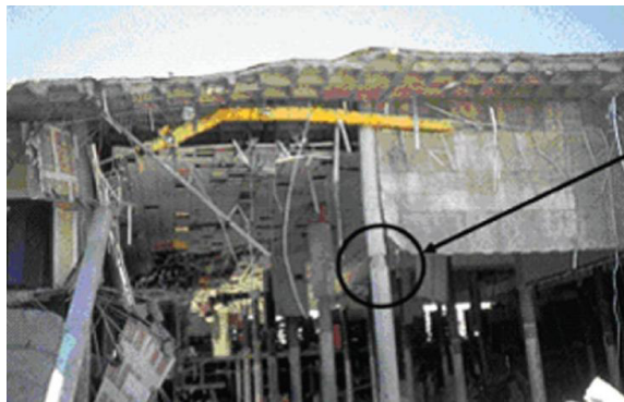
Figura 10. Falla por punzonamiento (Journal of engineering and technology).
