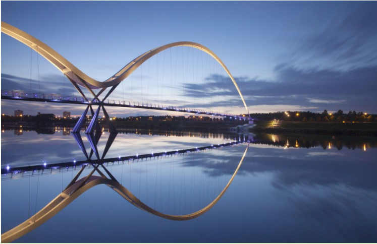
Figure 6. Infinity Bridge, Stockton-on-Tees, England.
