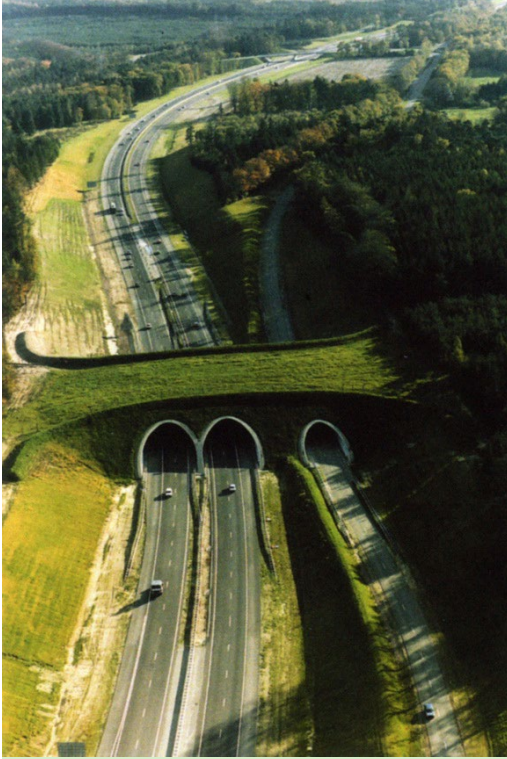
Figure 3. The Netherlands. Ecoduct over Highway A50.
